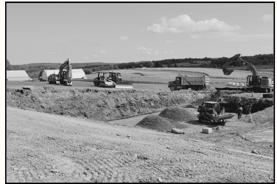
Above: Site preparation is underway for the construction of a new short-term manure storage facility.
